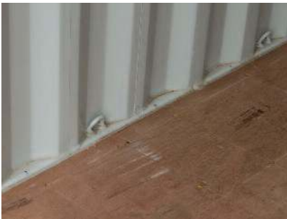
Container lashing points
